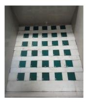
Figure 2: Pit after placing Dynemech Insulation Sheet and Filler Foam.
